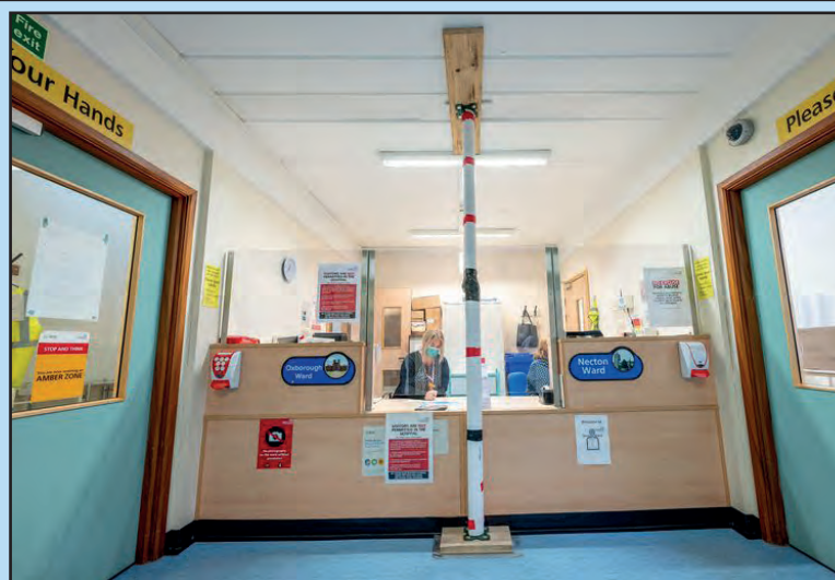
Thousands of metal props hold up QEH Kings Lynn until it's eventually rebuilt
